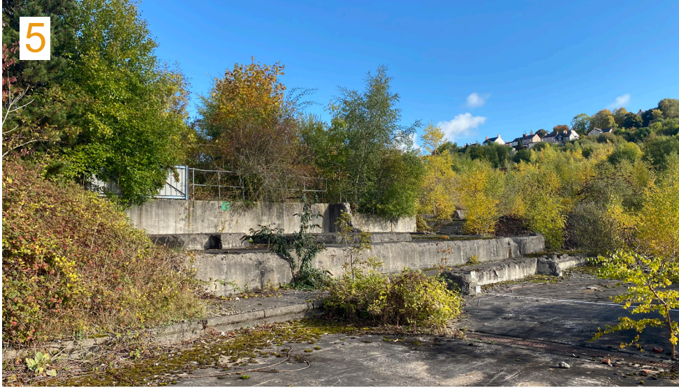
5. Remnant of the former industrial use. Existing reinforced concrete slabs and retaining walls
