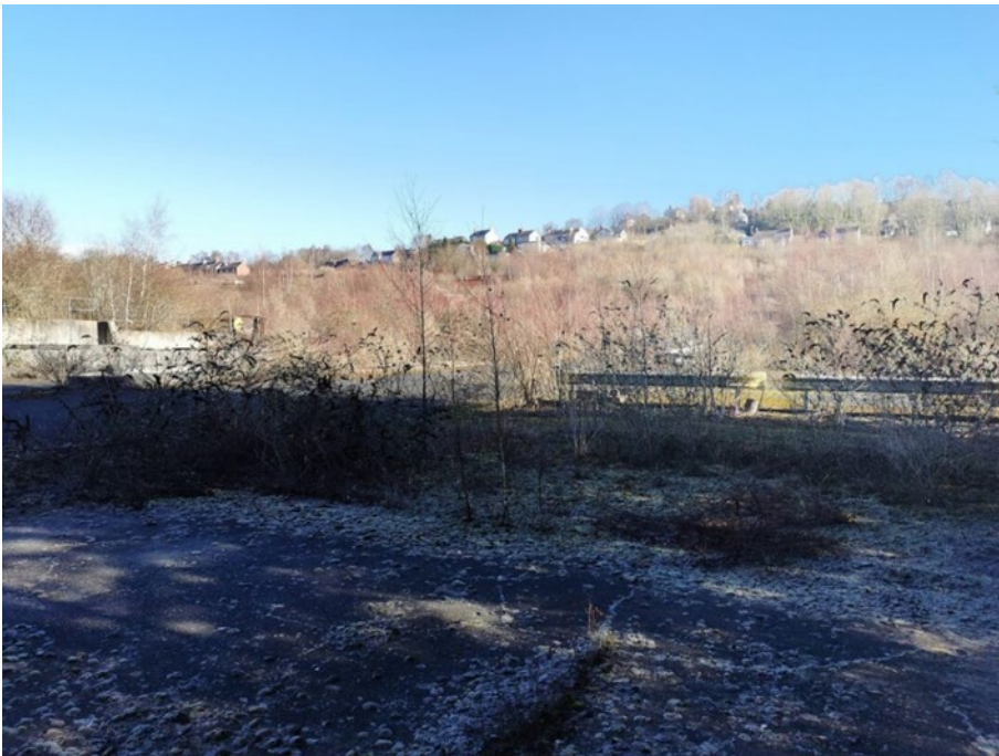
Plate 5: Demolished 20th-century industrial buildings in southern part of Site, looking north-east to residential development on the ridge at Cefn Mawr
