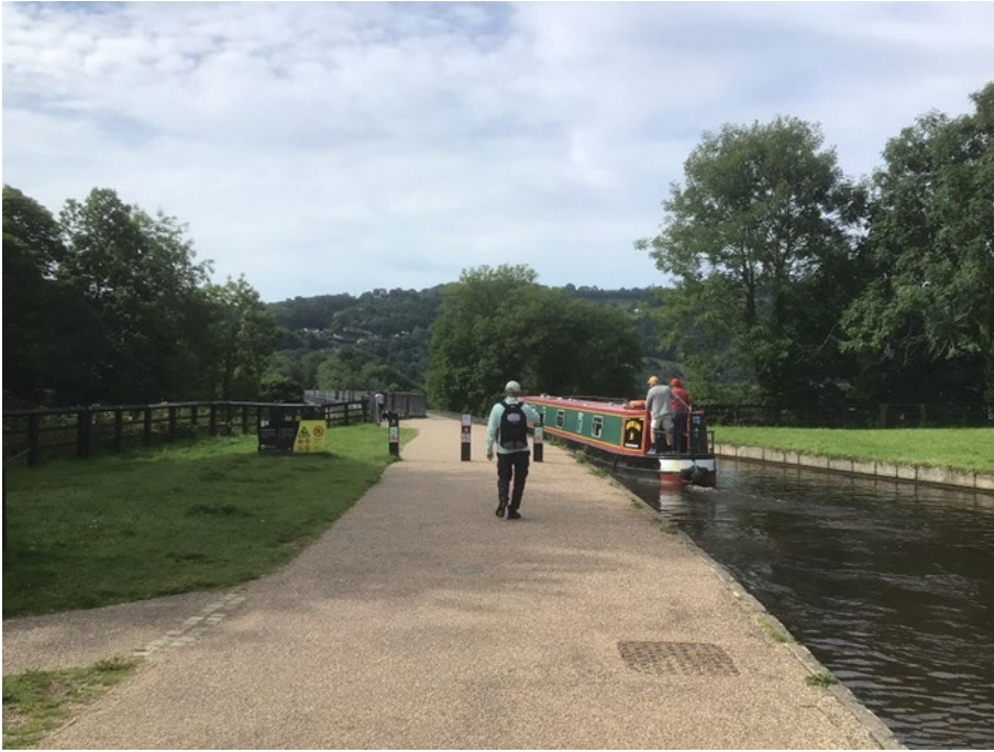
Plate 36: View south along canal towards Pontcysyllte Aqueduct (summer view)
