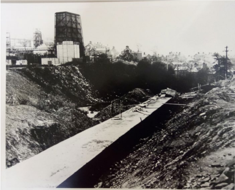
Plate 22: 1950s photo of the culverting of the Tref-y-nant Brook, exact location unknown (possibly to the south of the Site looking towards Cefn Mawr – photo courtesy of Ian Biggs)
