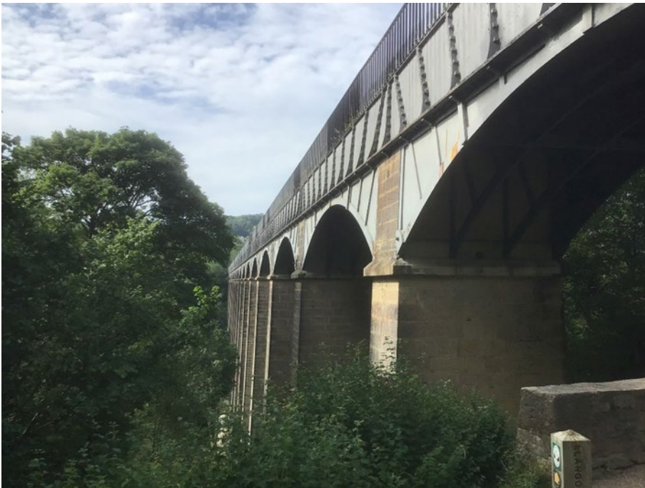
Plate 37: View of Pontcysyllte Aqueduct from PRow, looking south (summer view)
