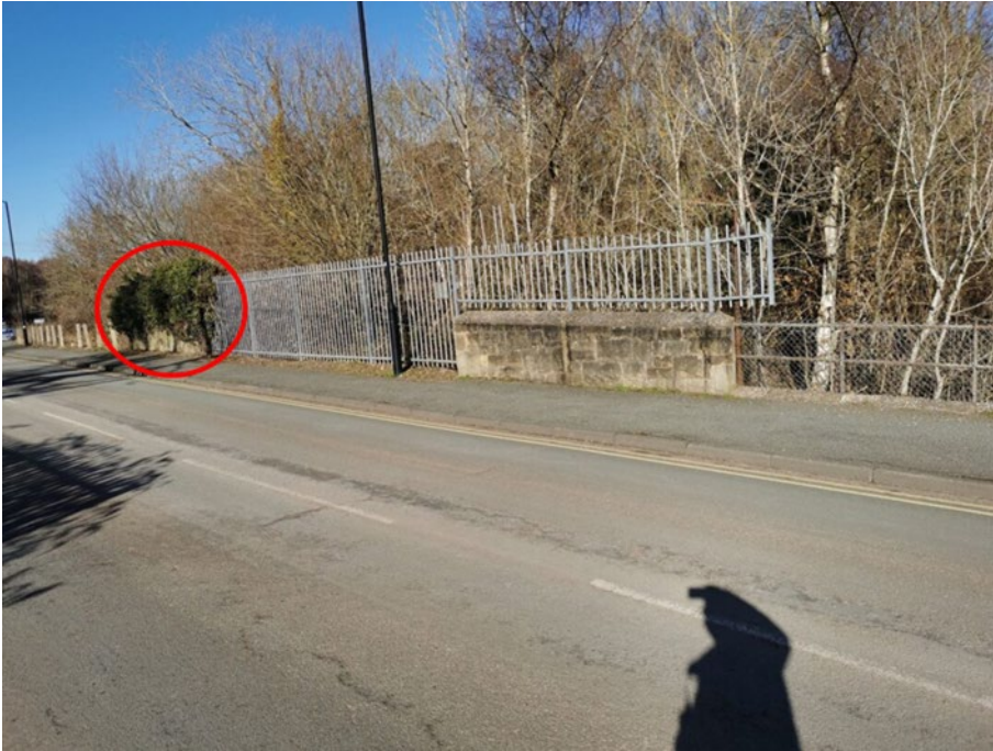
Plate 28: Queen St looking north, 20th-century overbridge in centre and abutment wall of 19th-century canal overbridge circled on left (the wall is located along the Site boundary)
