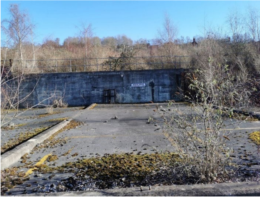
Plate 4: Demolished 20th-century industrial building in south-eastern part of Site, looking east
