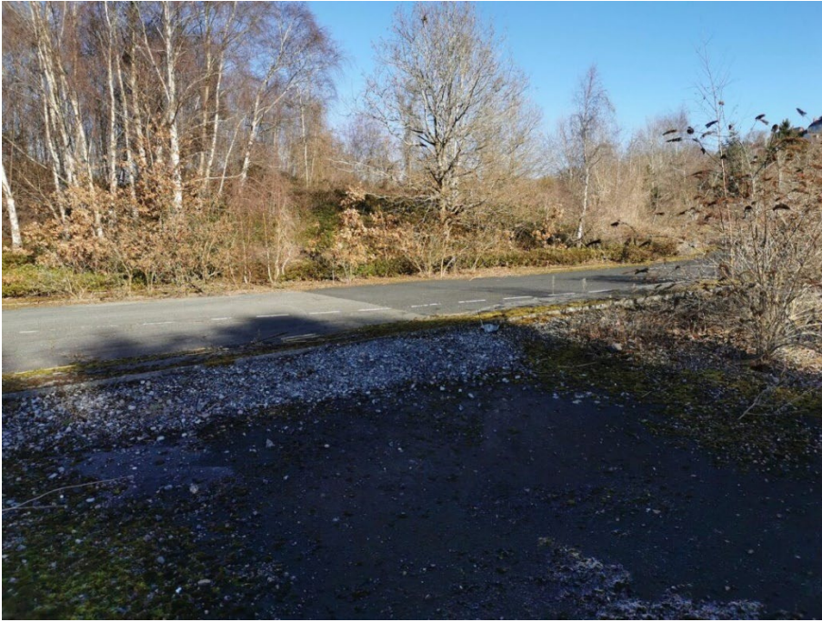
Plate 8: Internal access road within south-western part of Site, looking north
