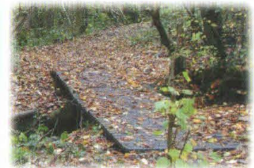
Bridge over culvert
