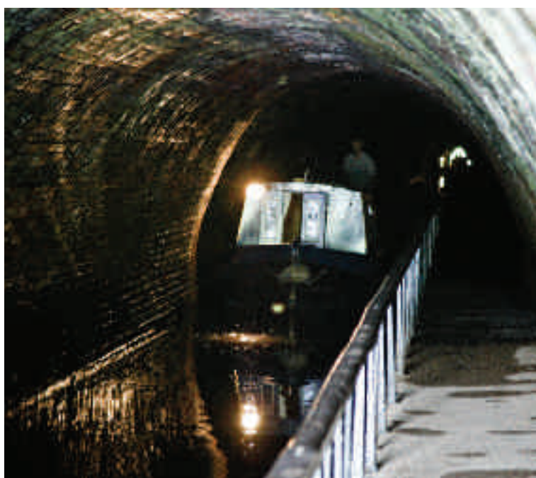
Whitehouses Tunnel, showing the path that permitted continuous towing by horses, now enjoyed by visitors.
